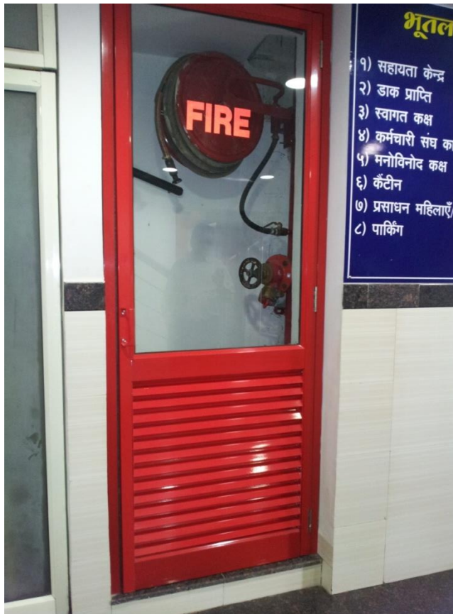
Landing Hydrant Installation
